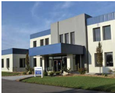
Plant I Administration Building (1-271A)
