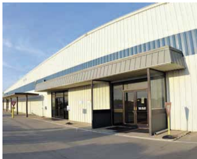
Industrial Park Building 3 (3-1900)
