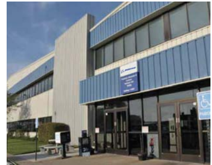
Strut-Nacelle Building - East (1-198D)
