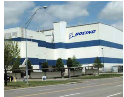
Manufacturing Process Facility (2-278M)
