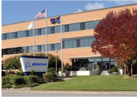
Administration Bldg/Plant II Entrance (2-270A) Check-in for badging.
