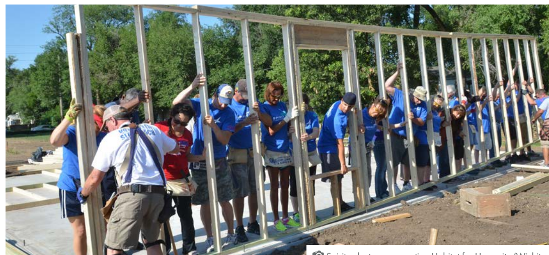
📷 Spirit volunteers supporting Habitat for Humanity (Wichita, KS).
